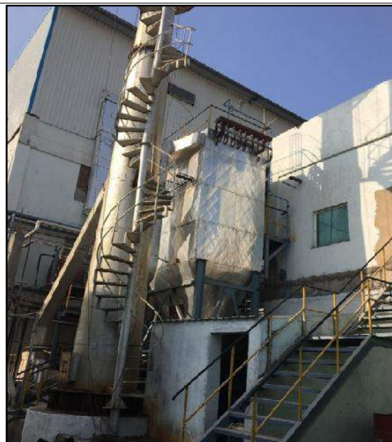
Bag filter attached with boiler stack
