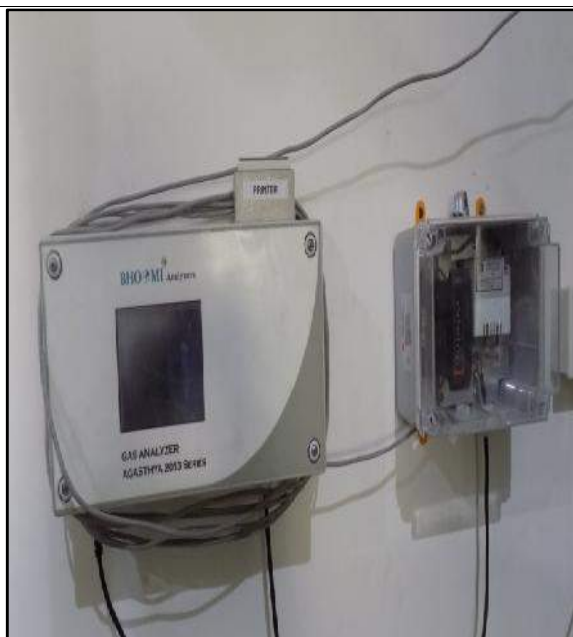
Boiler SPM Monitoring Panel
