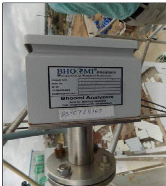
Boiler Stack Monitoring Sensor
