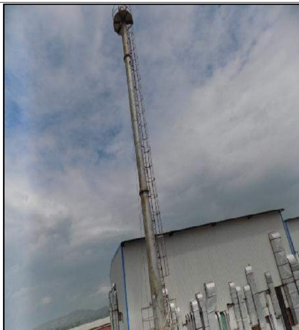
Adequate height provided to boiler stack
